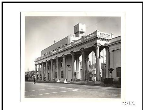
MGM's Colonnade entrance on Washington Blvd. built in 1915.
