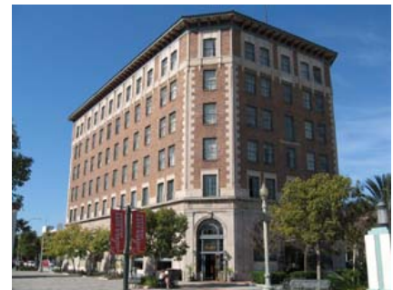
The historic Culver Hotel, built in 1924.
