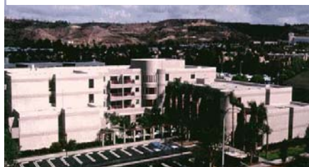
Culver City Rotary Plaza (looking east)
