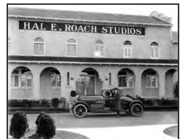
Hal E. Roach Studios, 1921 (Culver City Historical Society)
